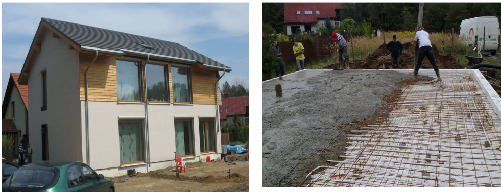
Fig. 1. Passive house in Boruszowice (left) and slab on grade during construction (right)
